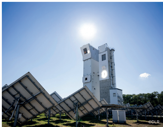
Solar Towers in Jülich
